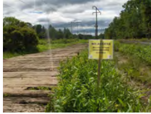
NO ACCESS – WETLAND/STREAM CROSSING MATS REQUIRED
